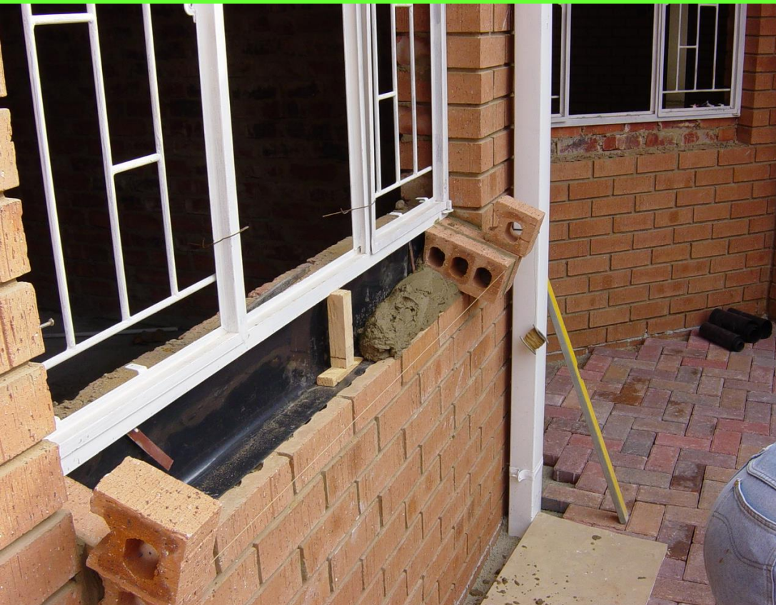
Fixing windows to openings
